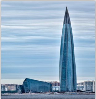
Gazprom Lakhta Center
